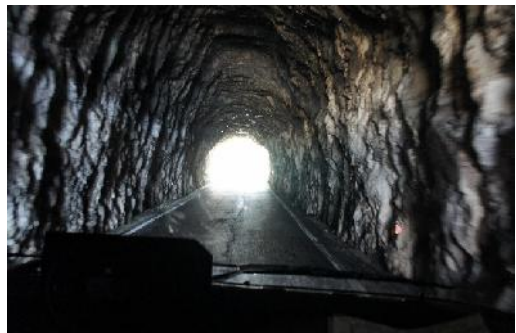
Rough dark tunnel on coast rd
