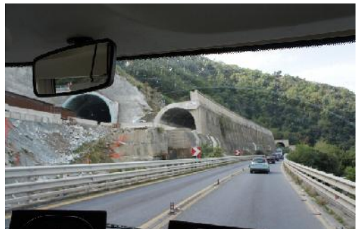
New tunnel construction on A3
